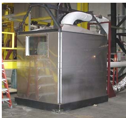
Figure 2-2 Technikon Research Foundry Emission Collection Hood
