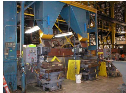
Figure 1 Osborn Molding Operation
