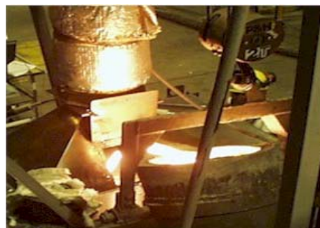
Pouring of Step Core Molds Through Opening in Collection Hood
