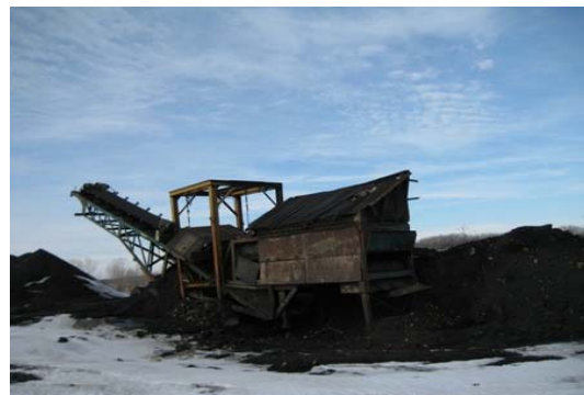
Figure 2. Machine that crushes and screens the core sand.
