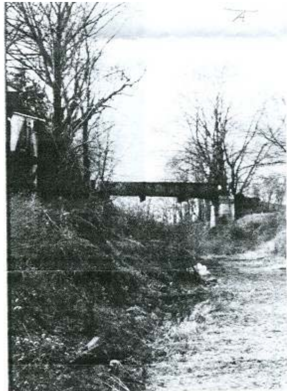
Photo 2: A view (looking west) of the old bridge crossing the abandoned railroad bed. The bridge was removed by Littco and an embankment was built up directly under its old location to support the portion of Bridge Street that now crosses the former railroad bed.
