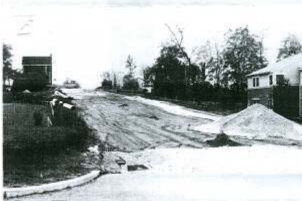
Photo 3: A view looking south along Bridge Street before its completion.
