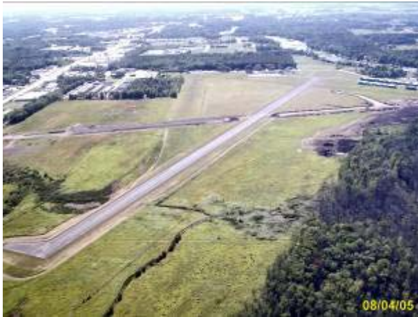
Photo 1: An aerial shot of the runway in construction.
