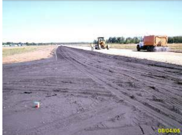
Photo 2: The runway in construction. Note the watering truck to the right.
