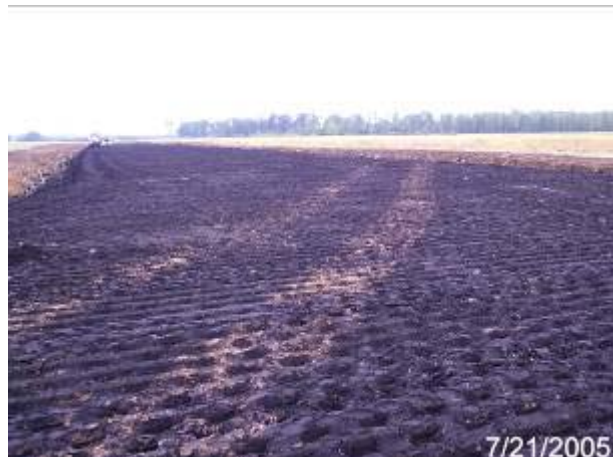
Photo 3: Foundry sand in place and compacted.
