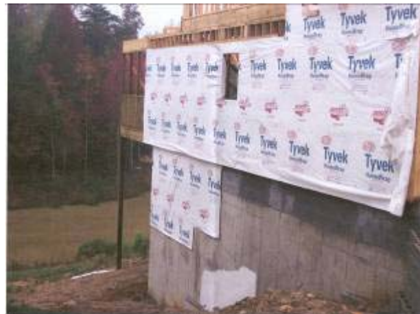
Photo 1: A view of one of the homes that used Eureka's sand as foundation fill. The building site was excavated down to stable ground, and then the foundry sand was used as fill to get the foundation back up to the necessary grade.
