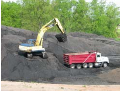
Figure 1. Transferring spent foundry sand to the construction site.
