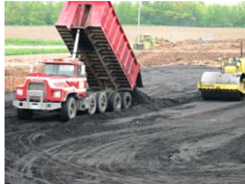
Figure 2. Compacting fill material at the project site.
