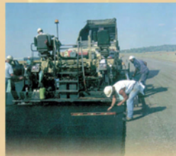
A consortium of West Michigan foundries reuses foundry by-products in asphalt paving and as a landfill liner cover.
