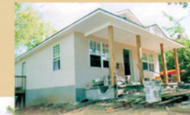
Wheland Foundry of Tennessee uses foundry sand mixed with cement and clay to make terra blocks. These blocks built this Habitat for Humanity home in Chattanooga.
